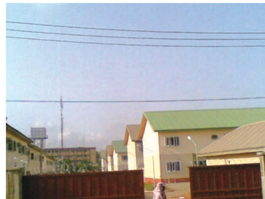
Figure 1 Gate House View of Estate
