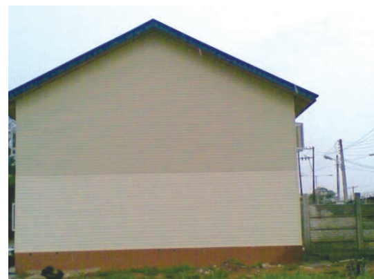
Figure 2 Side View of Estate With PVC Claddings
